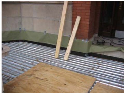
Installed Galvanized Steel Decking
