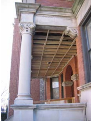
Removed and Replaced Ceiling Framing
