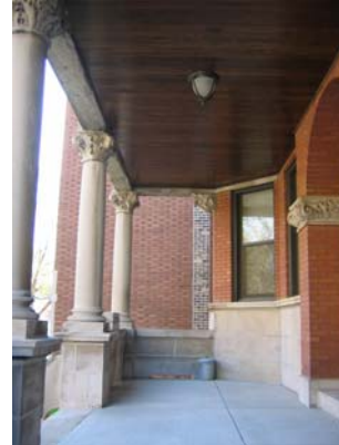
Poured/Finished Steel Reinforced Concrete Slab and Installed New Bead-Board
