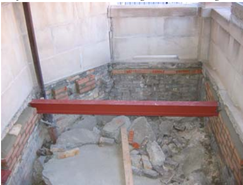
Repaired Masonry and Installed Steel Beams
